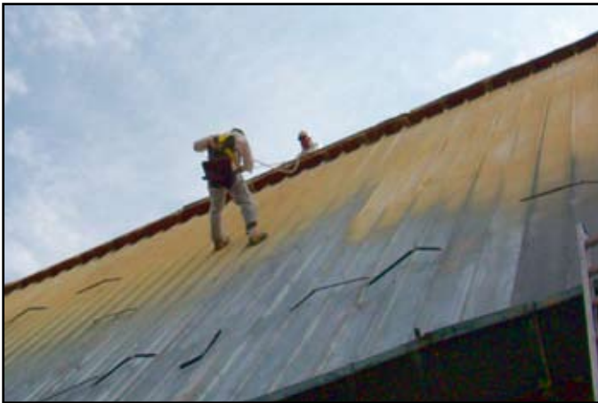
SPF to a vertical metal mansard.
