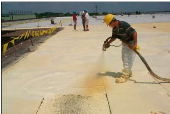
The SPF is fully adhered to the old roof system.
