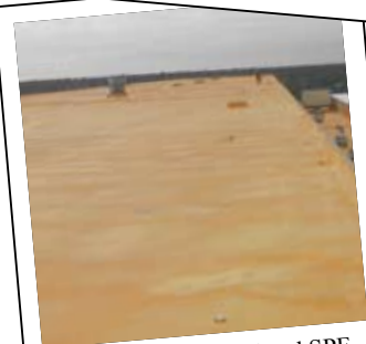
Overview of completed SPF
