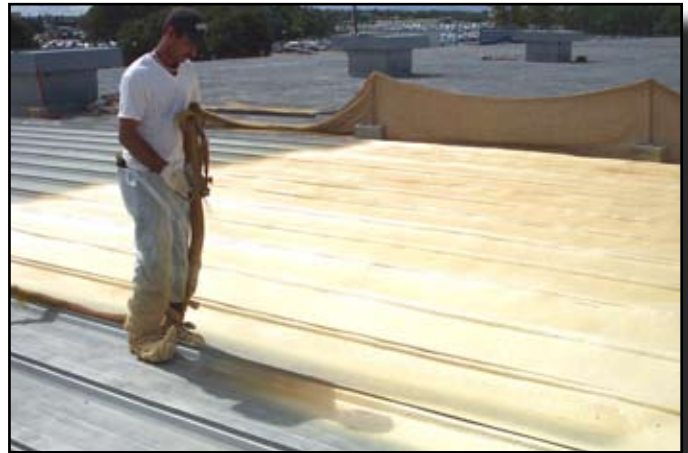
SPF over a metal roof system.
