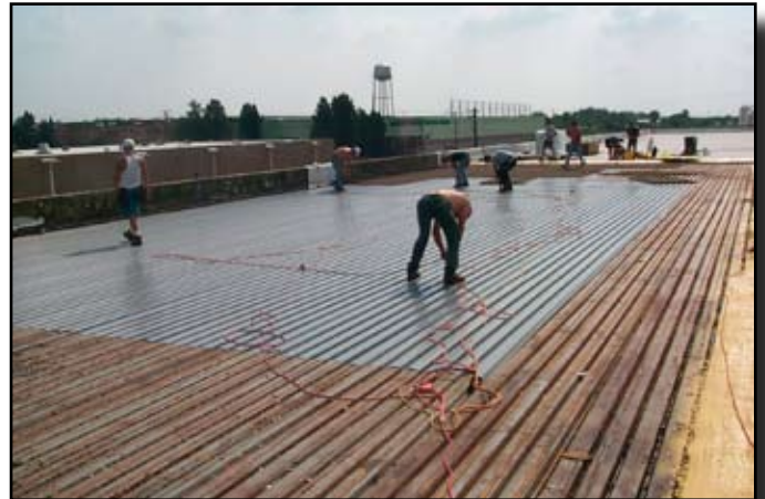
The completed metal deck area.
