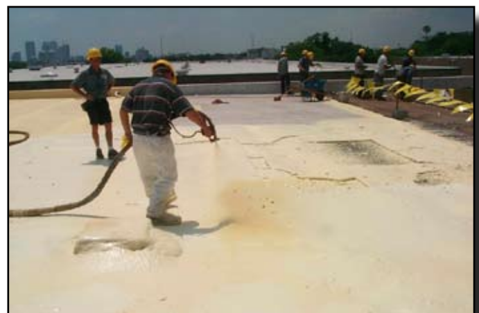
The SPF conforms to the contour of the surface to which it is applied, sealing all cracks and crevices.
