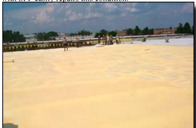
The completed SPF temporary roof system.
