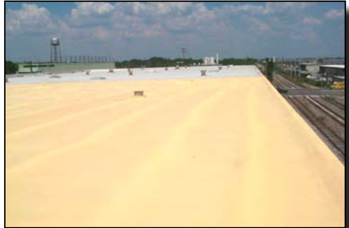
The SPF is fully adhered to the existing surface providing maximum “hold down” capabilities.
