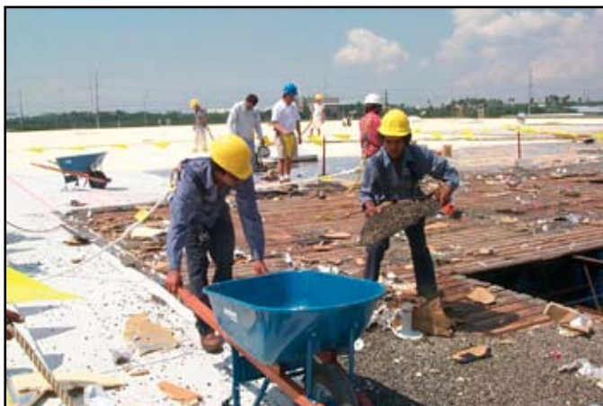
Debris is removed from the rooftop.
