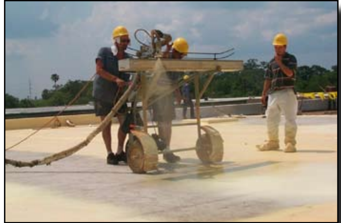
SPF over a single ply membrane.
