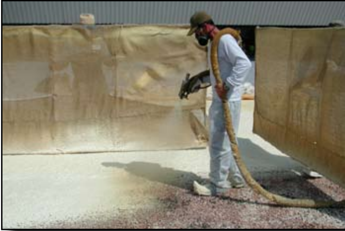
SPF over a built-up gravel (BURG) surfaced roof.
