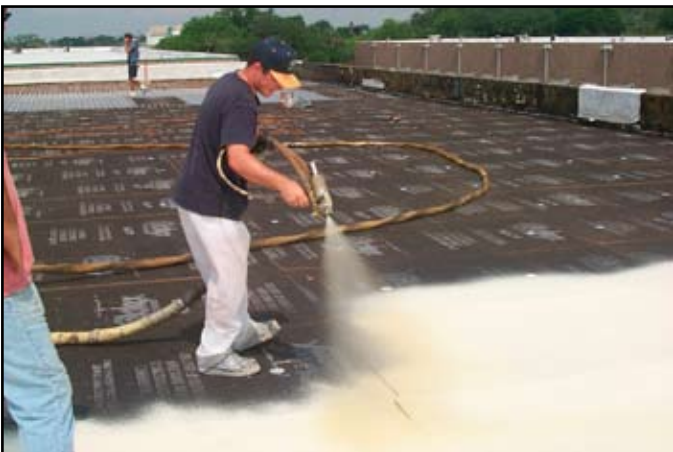
SPF is spray applied directly to the insulation board.
