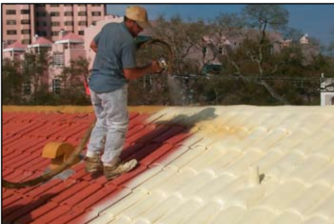
SPF over a concrete tile system.
