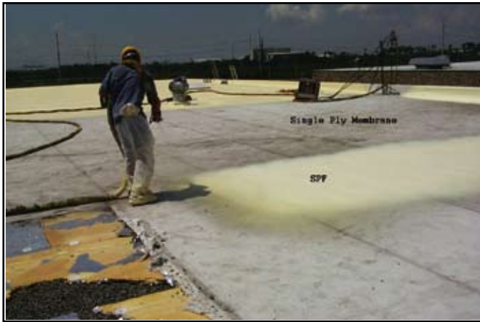
SPF is spray applied directly to the existing single ply membrane.
