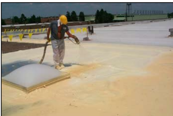
The SPF is quickly applied and becomes completely watertight within minutes.
