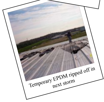
Failed Temporary EPDM
