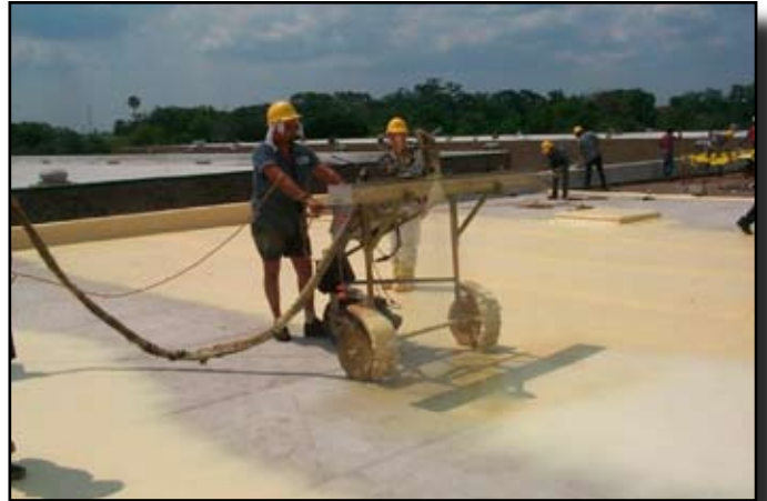
On large open areas, robotics can be utilized for maximum production.
