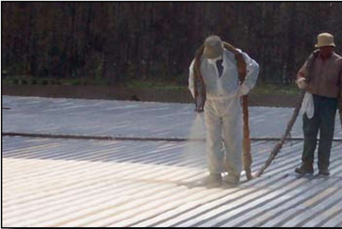
SPF sprayed directly to a corrugated metal deck.
