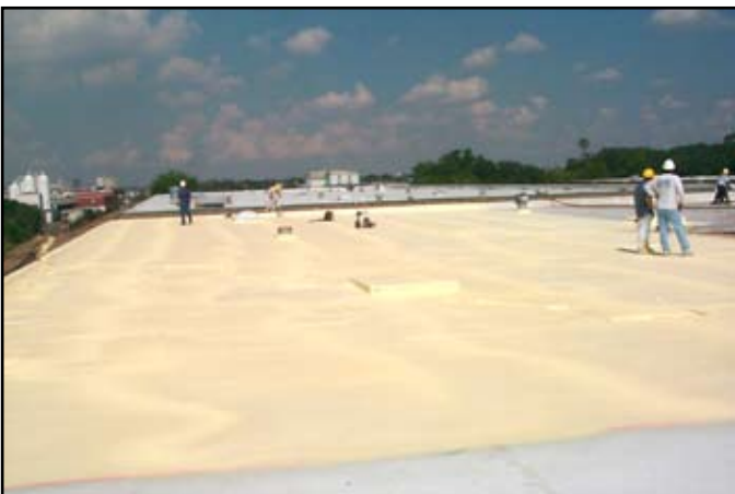
The completed SPF temporary roof system.
