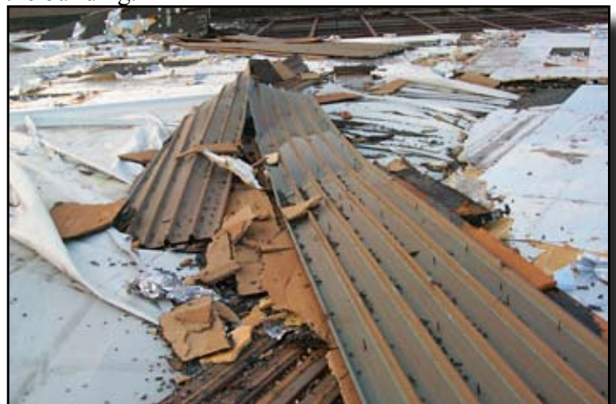
Sections of metal deck is scattered around the roof.
