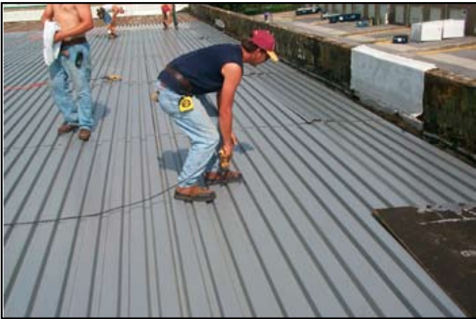
Metal deck is installed and screwed to the existing structural purlins.
