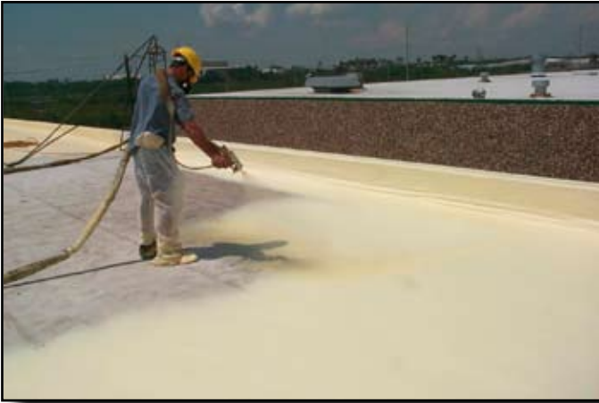
A 1" thick, seamless waterproofing "blanket" adheres to everything.
