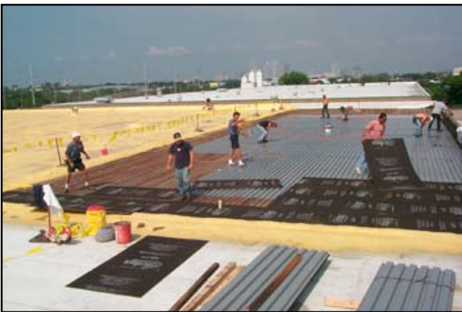
Insulation board is applied to the new metal deck.
