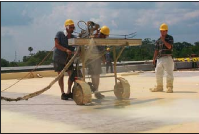
SPF is spray applied using robotic technology.
